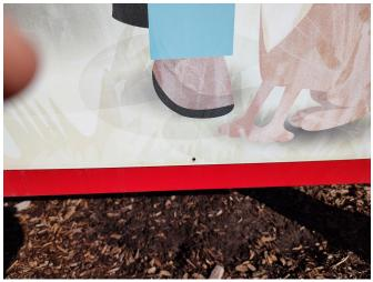
Loose hardware on one of the barriers (CPSC 2.5.2)(Priority 3 Hazard -Hardware resecured by Keith Kroening on 3/23/2024)
